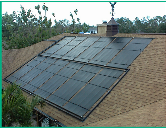
6 (4x10') & 6 (4x8') Vortex double row roof installation
