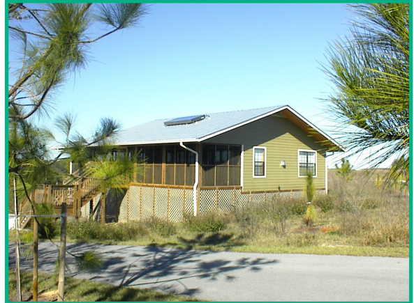
State park cabin PT installation
