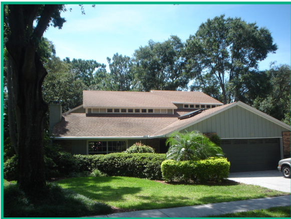
Front of house PT solar hot water installation
